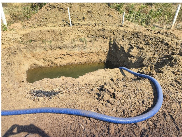
Water stored in the pond constructed under the project used for irrigation in village Tungburu, East Singhbhum
